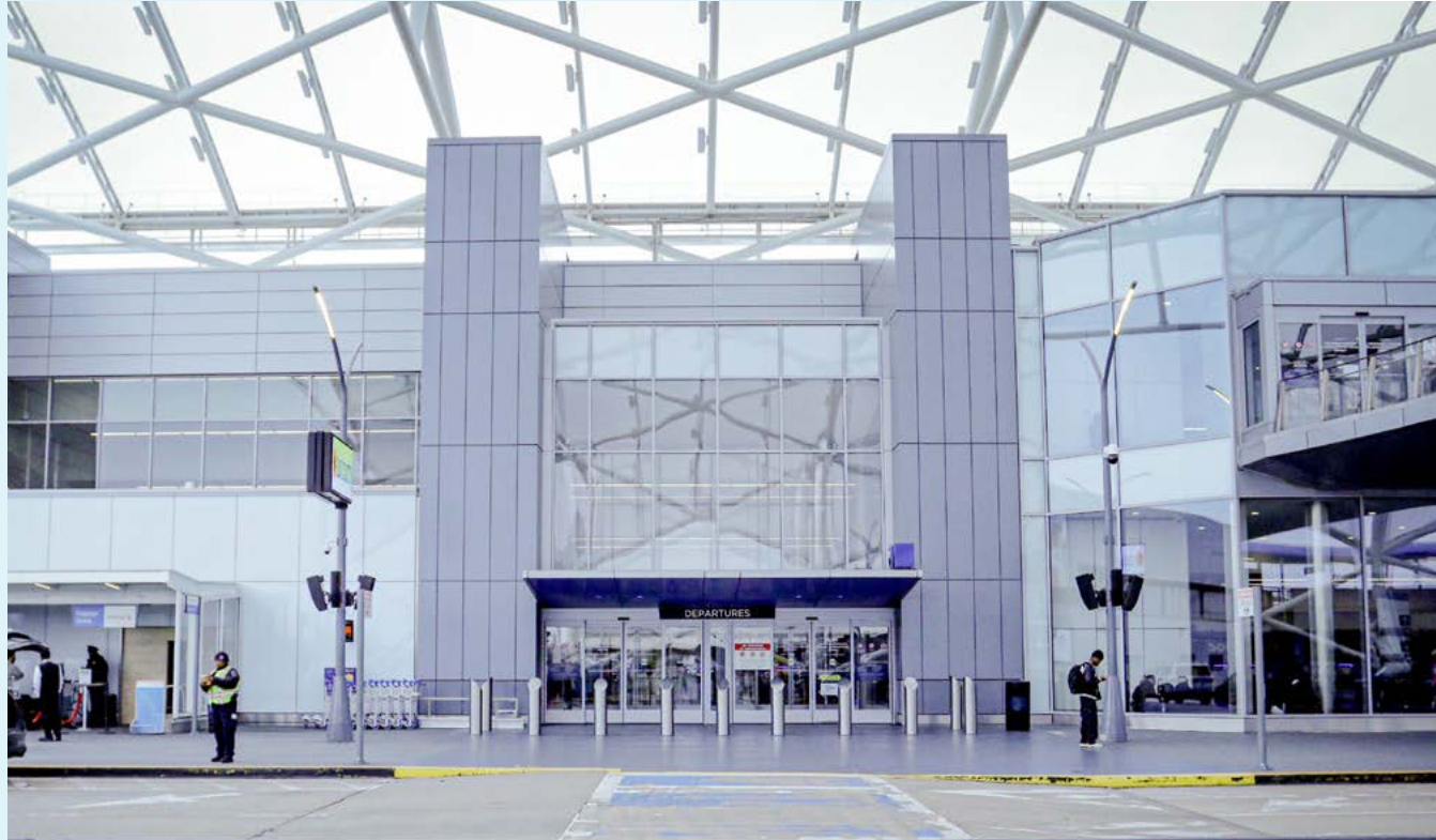
Hartsfield-Jackson Atlanta International Airport Terminal 2025
